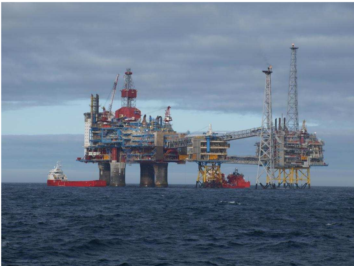
Fig. 19: CO 2 injection/CH 4 production platforms located at the Sleipner Vest gas field.
